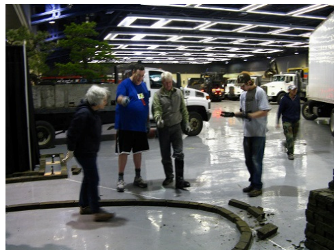
Laying out the first row is the most important.
