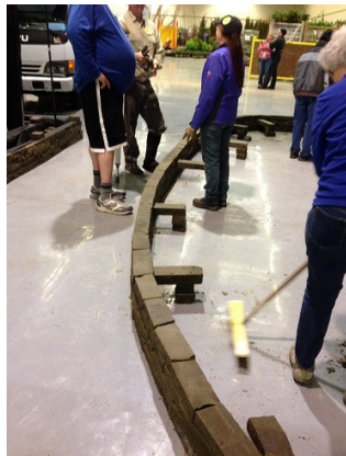
Building the knee braces to support the rock wall.
